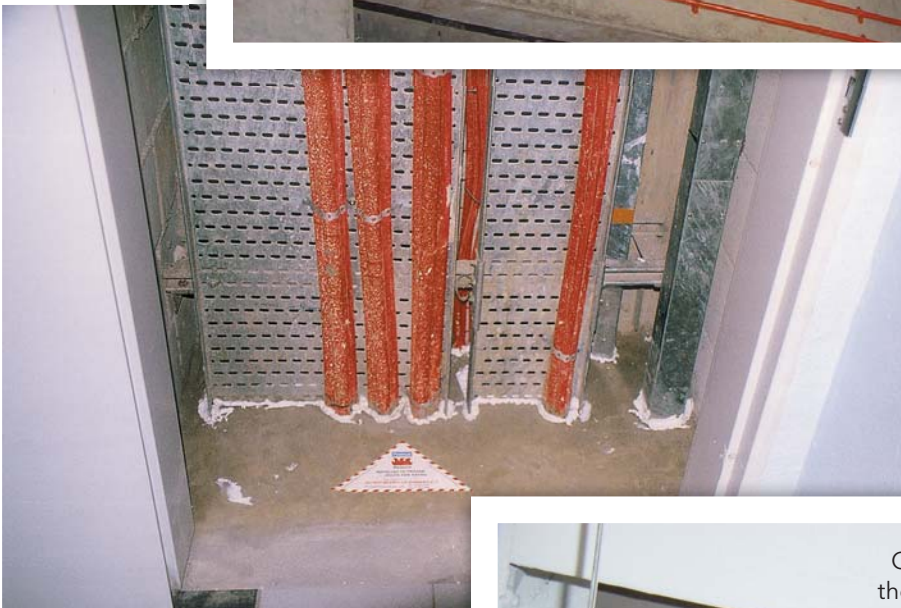
Electrical cables penetration seal through masonry slab inside the control room of Menara Great Eastern, Kuala Lumpur, Malaysia
