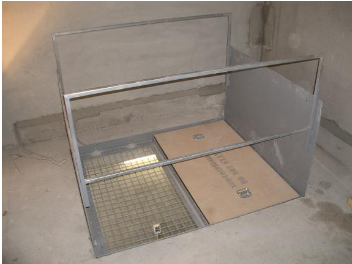
Fire rated lift motor room hatch installed – 1 lid open
