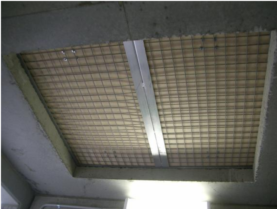
Fire rated lift motor room hatch installed—underside view
